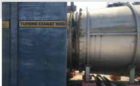
A fabric expansion joint from EagleBurgmann in a similar application in India.
