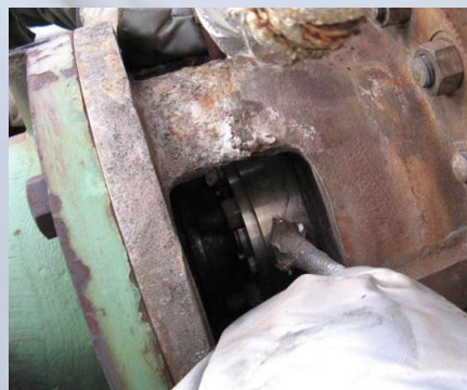
The sulfur transfer pump after retrofitting to EagleBurgmann SulfurAce: no leakage, no contamination
